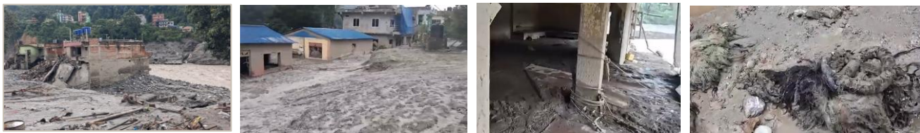
▲ Debris-flow damage in the town centre (Bidur, photo by our local partner). Along the river, mud reached rooms on the second floor and above, and a drowned buffalo was washed ashore.
